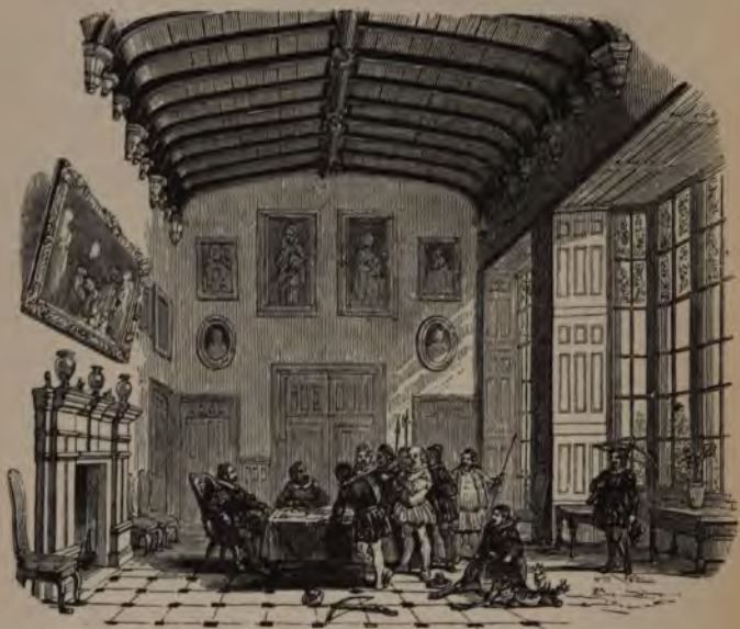
Hall of Charlecote.
